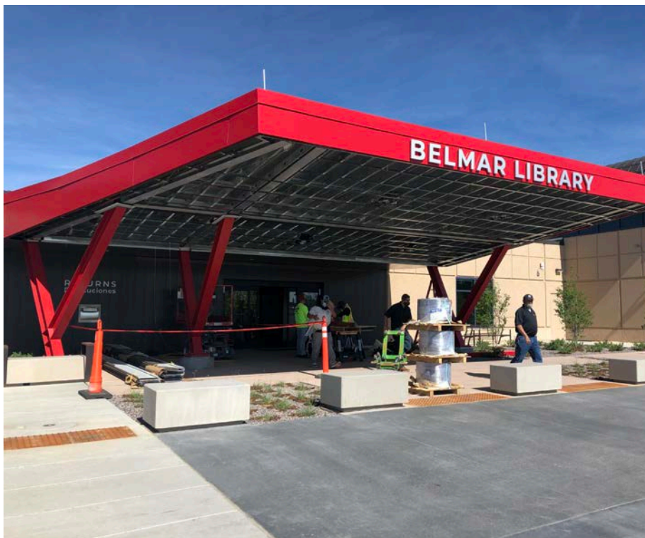
Exterior Canopy – Re-work of underside of canopy ceiling
