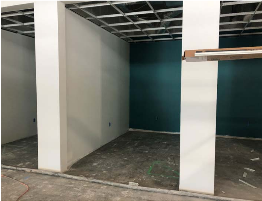
Study Rooms – ceiling grid and paint complete
