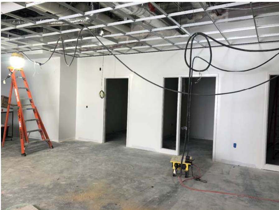
Ceiling Grid and Staff Offices
